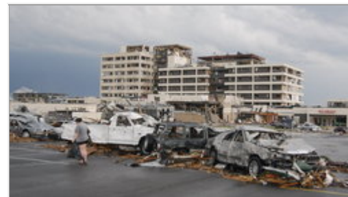
Damaged vehicles litter the parking lot of St John's Hospital in Joplin, Missouri, after a tornado hit the Southwest Missouri city on Sunday, May 22. According to reports, the tornado hit the hospital head-on. [Mike Gullett/AP, Photo]
