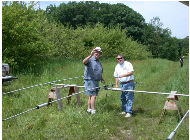
Above Peter N1ZRG and Les N1SV assembling the yagi that will go on the Beltronics trailer tower.
