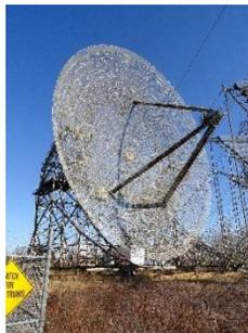
Despite some lingering SWR issues that kept his power down to well less than ten watts at the antenna feedpoint, Will racked up four CW, five SSB, and eighteen JT65-B QSOs during the weekend. Gain (42dB) helps!
