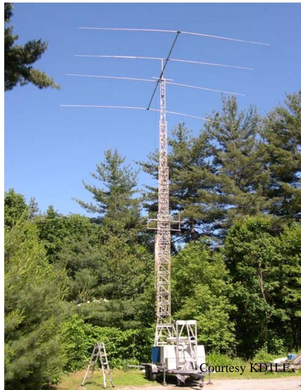
Since the antenna boom of the 20 meter antenna is too long to be put on the mast when the tower is horizontal it had to be mounted in two pieces. The
