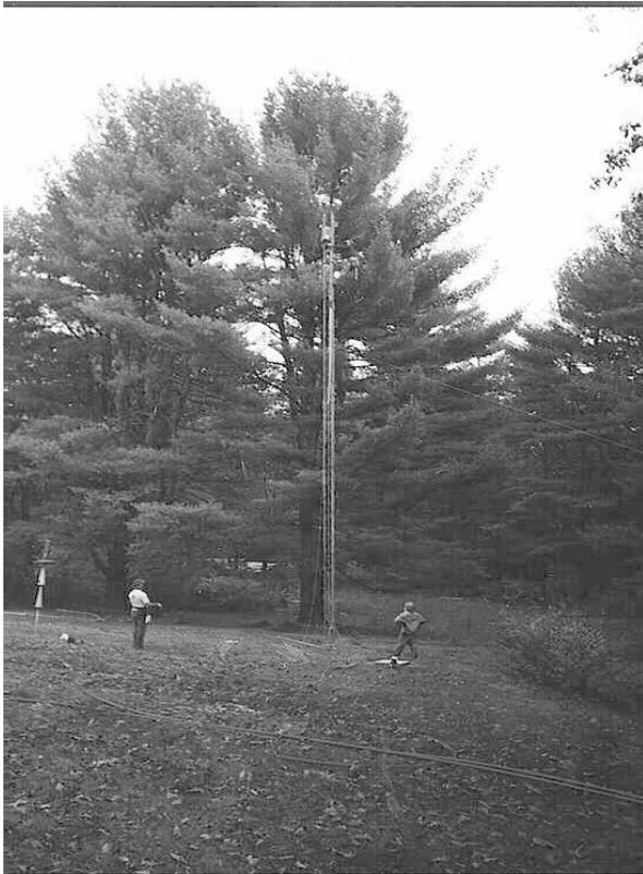
top. The second day we put up sixty feet of tower bringing the tower to its final one hundred foot height. The next picture is Ralph and Stan struggling to make two of those ornery tower sections fit together. On the third day we straightened the tower, tensioned the guys, mounted the mast and
